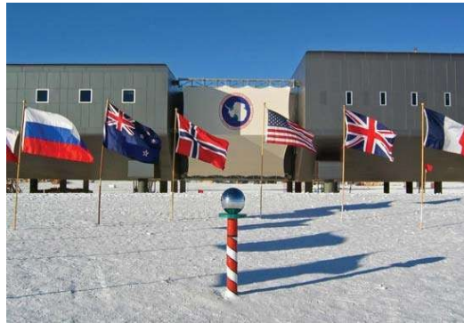
Amundsen-Scott South Pole Station, South Pole, Antarctica
